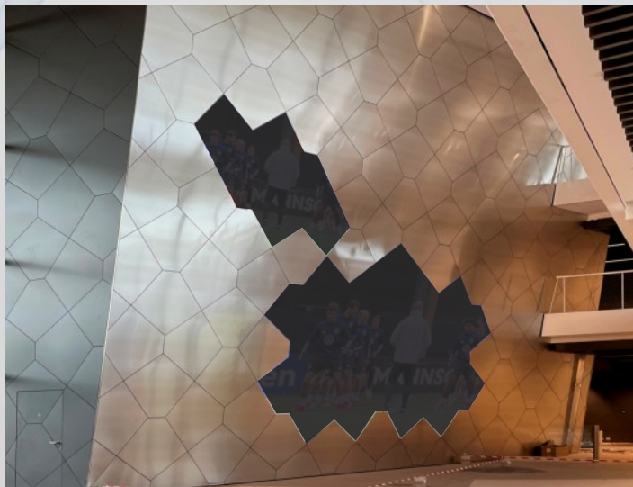
Aluminum facade with LED Wall
